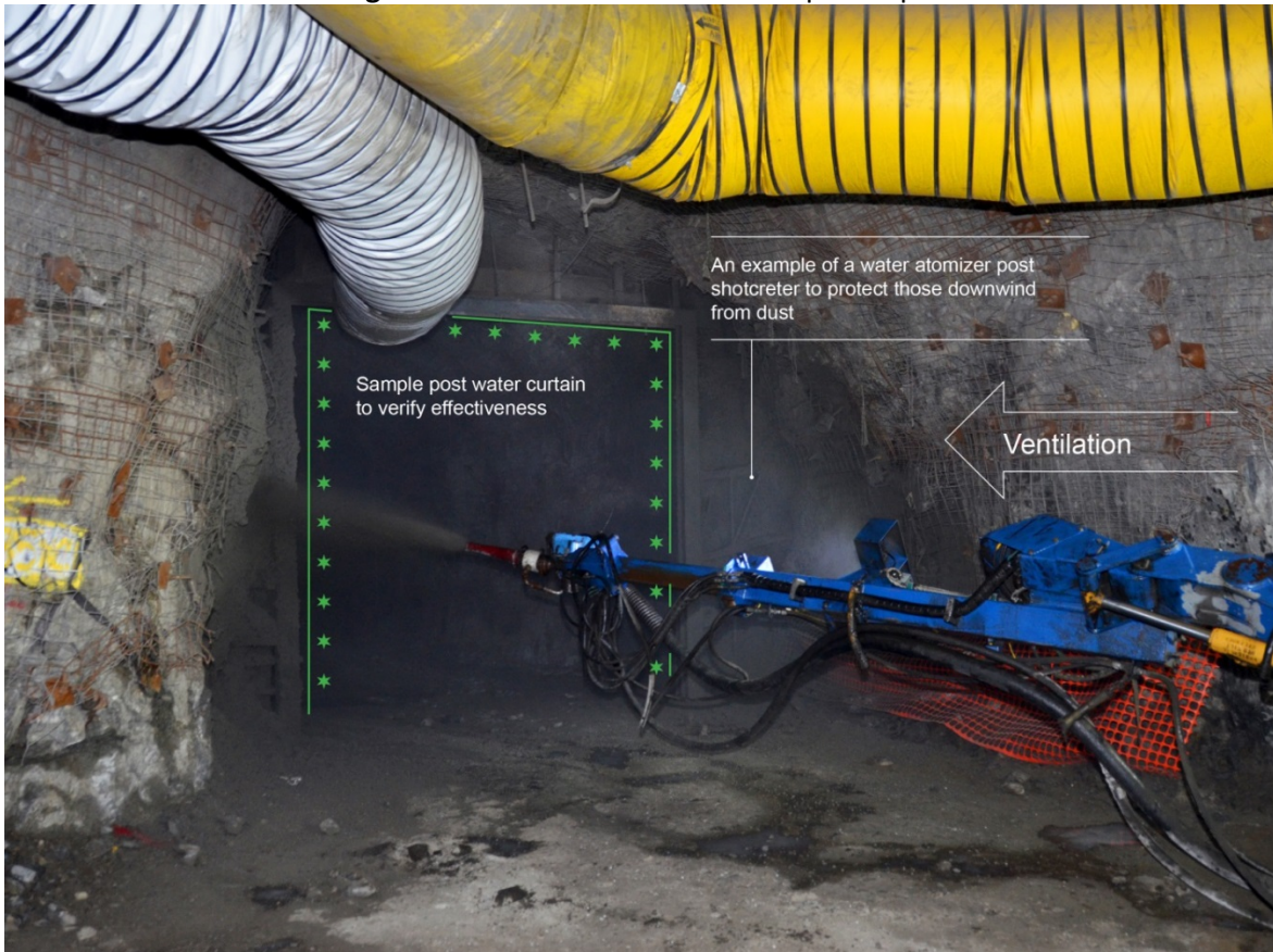
Figure 5 – Shotcrete Atomizer Set-up Example
