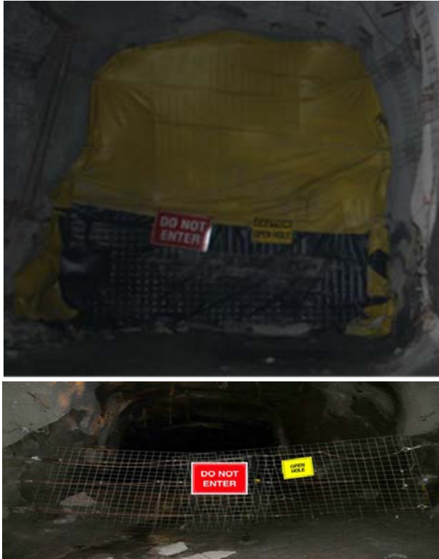
Figure 3 - Examples of no entry type barricade.
