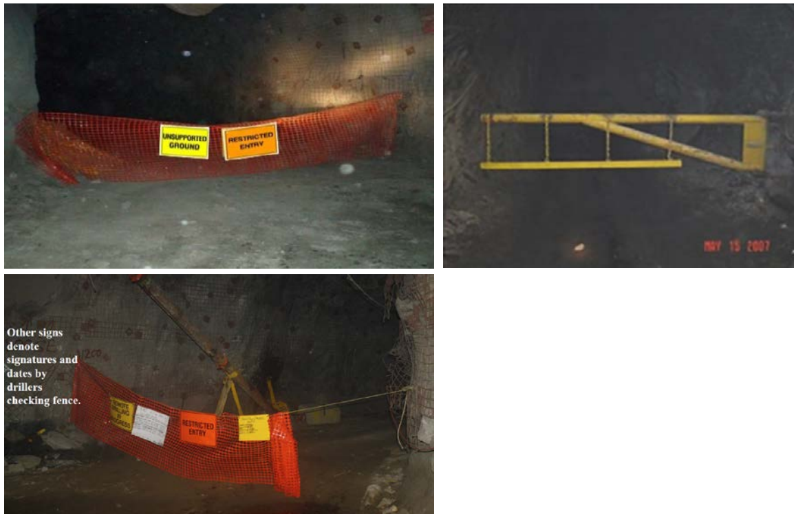
Figure 4 - Examples of restrictive warning type barricade.
