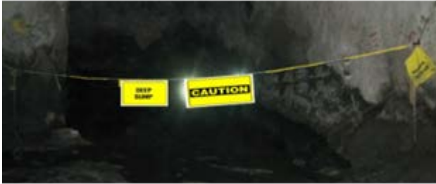
Figure 5 - Example of cautionary type barricade.
