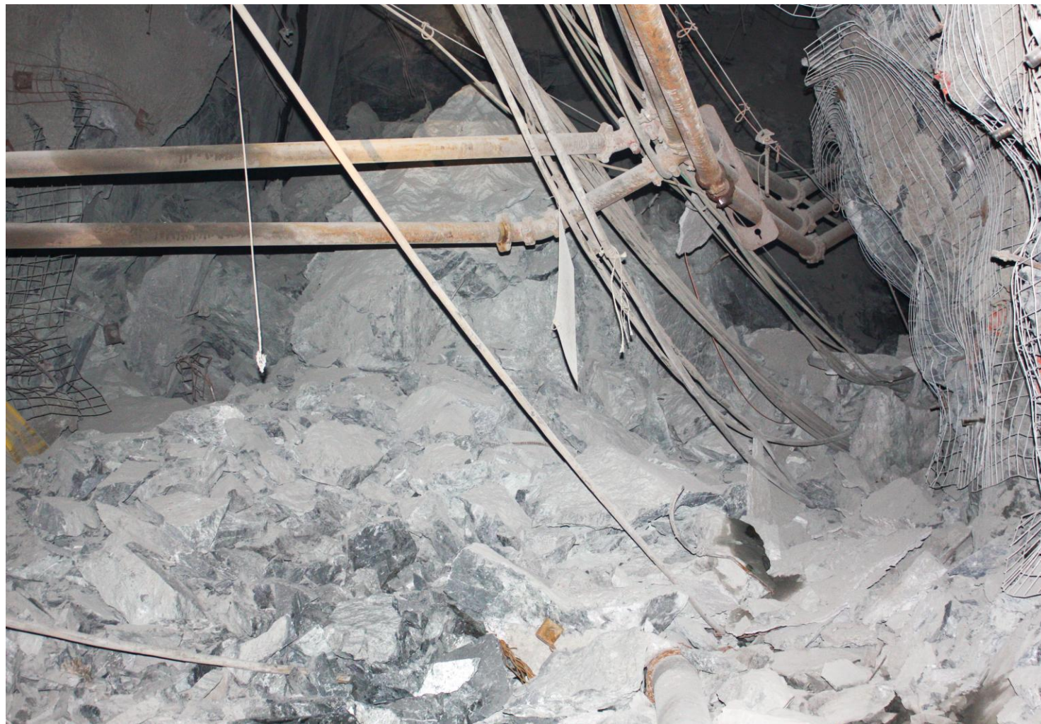
Main (footwall) drift damage from M n 3.8 Seismic Event
