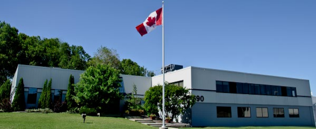
WSN Health and Safety Training Centre and Ontario headquarters in North Bay
