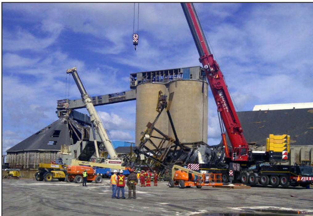
Four cranes were required to lift the wreckage of a loading boom, above, but rescuers still had to get close to clear debris and cut through tubular steel and angle bar.
