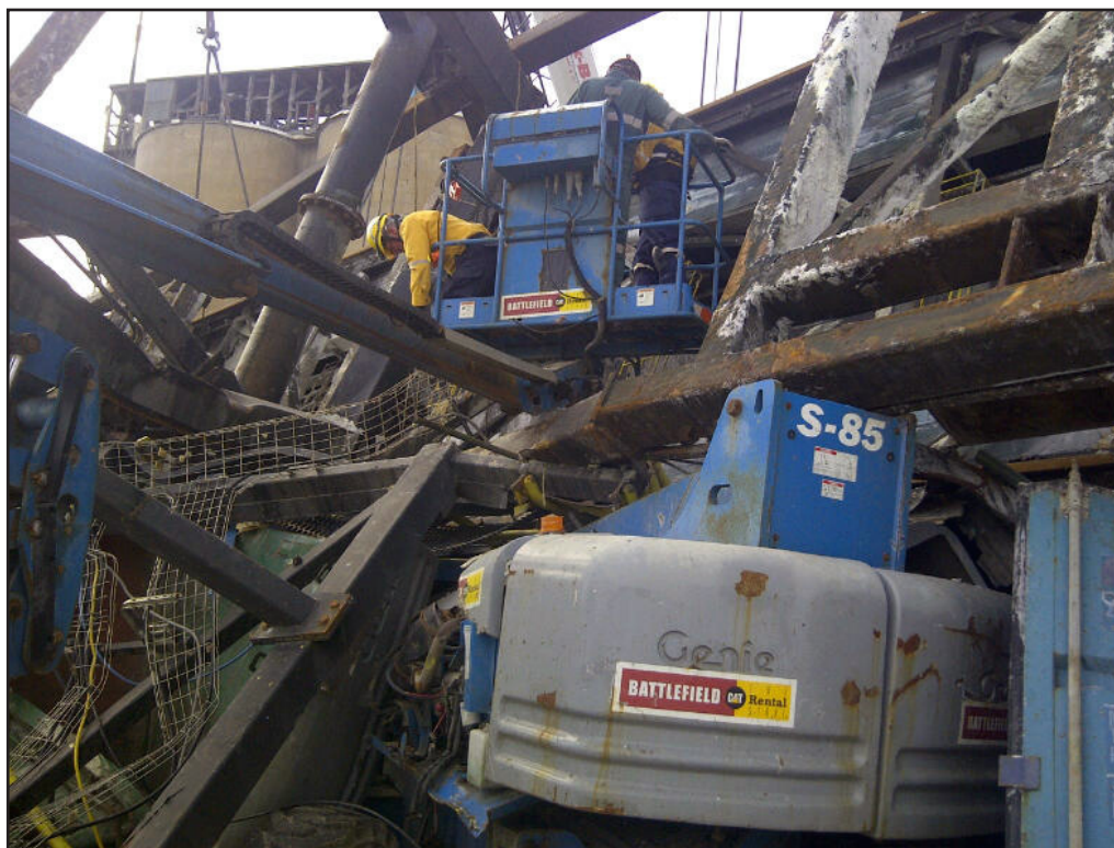
Four cranes were required to lift the wreckage of a loading boom, above, but rescuers still had to get close to clear debris and cut through tubular steel and angle bar.
